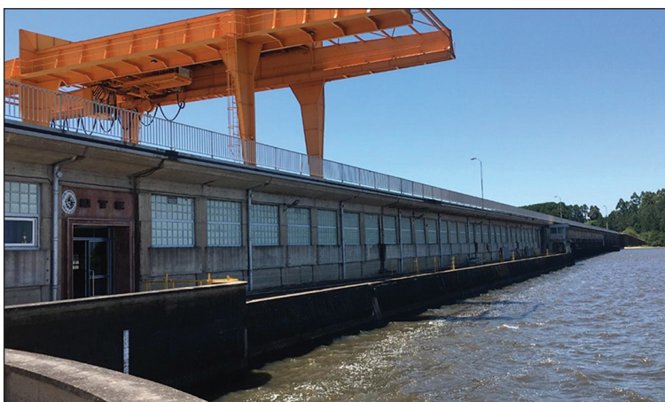
The 105 MW Baygorria hydro plant in Uruguay.
